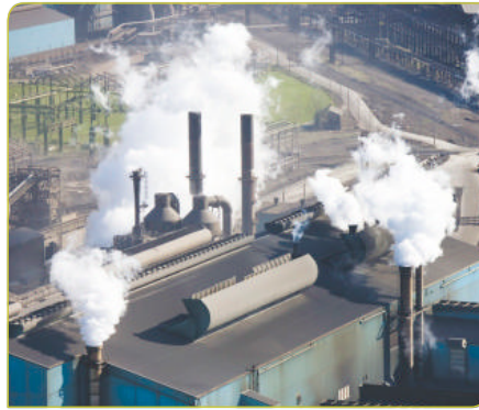
Aerial view of factory in Gary, Indiana.
